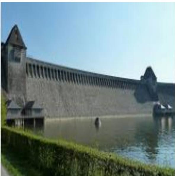
The Mohne Dam had two towers at either end, as seen in the picture. To ensure that the bomb was released at the correct distance of 450 yds from the target, a simple triangular wooden sight with two vertical nails was devised, through which the aimer looked. When the dam lined up with the two nails, the bomb was released.
